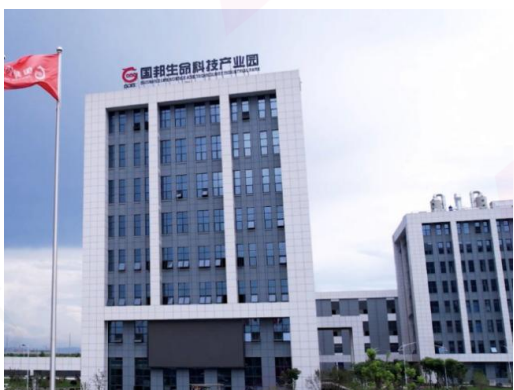
上虞国邦医药生命科技产业园外墙防水装饰，绍兴，浙江 Shangyu Guobang Pharmaceutical Life Science Industrial Park, Exterior Wall Waterproof&Decoration, Shaoxing, Zhejiang
