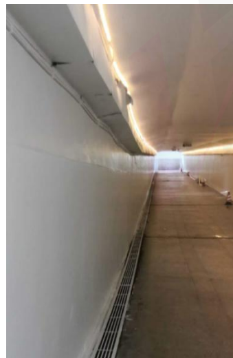
地下人行通道内墙防水装饰, 曲靖, 云南 Underground Pedestrian Passage Interior Wall Waterproof&&Decoration, Qujing, Yunnan
