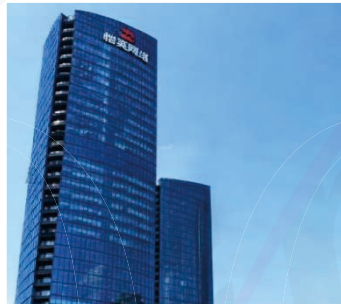
恺英网络大厦幕墙工程, 杭州, 浙江 Kaiying Network Building, Curtain Wall Project, Hangzhou, Zhejiang
