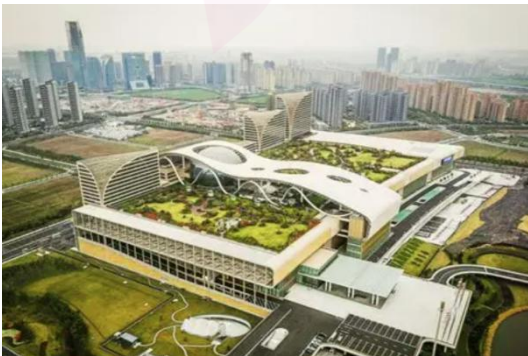
杭州国际博览中心钢结构防腐装饰, 杭州, 浙江 Hangzhou International Expo Center, Steel Structure Anti-corrosion&Decoration, Hangzhou, Zhejiang
