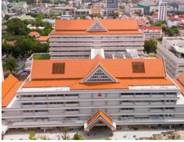
玛霍索综合医院幕墙工程, 老挝 Mahosot General Hospital, Curtain Wall Project, Vientiane, Laos
