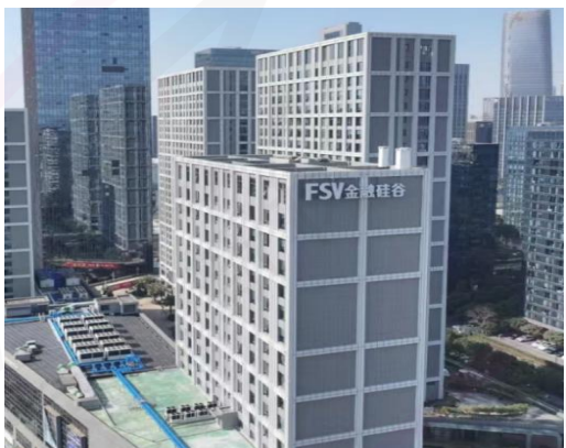
金融硅谷中心外墙防水装饰，宁波，浙江 Financial Silicon Valley Center, Exterior Wall Waterproof&Decoration, Ningbo, Zhejiang
