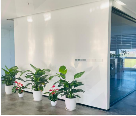
浙江凌志新材料办公大楼内墙防水装饰, 杭州, 浙江 Zhejiang Liniz Advanced Material Office Building Interior Wall Waterproof&&Decoration, Hangzhou, Zhejiang
