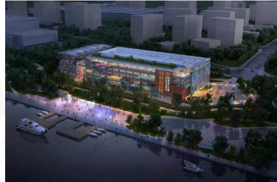
世博园宋城演艺中心钢结构防腐装饰, 上海 Songcheng Performing Arts Center in Expo Park, Steel Structure Anti-corrosion&Decoration, Shanghai
