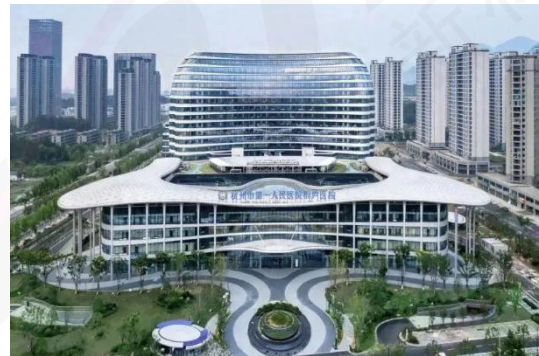
杭州第一人民医院桐庐分院钢结构立柱防腐装饰, 杭州, 浙江 Tonglu Branch of Hangzhou First People's Hospital, Steel Structure Column Anti-corrosion&Decoration, Hangzhou, Zhejiang
