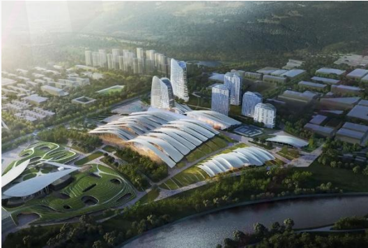
“两山”国际会展中心钢结构防腐装饰, 湖州, 浙江 "Two Mountains" International Convention and Exhibition Center, Steel Structure Anti-corrosion&Decoration, Huzhou, Zhejiang
