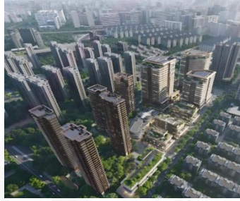
长风宸嘉地产项目幕墙工程, 上海 Changfeng Chenjia Real Estate Project, Curtain Wall Project, Shanghai
