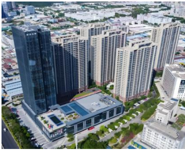
汕尾星合里写字楼项目幕墙工程, 汕尾, 广东 Shanwei Xingheli Office Building Project, Curtain Wall Project, Shanwei, Guangdong
