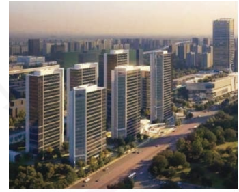
滨江 T-ONE 潮博中心幕墙工程, 杭州, 浙江 Binjiang T-ONE Chaobo Center, Curtain Wall Project, Hangzhou, Zhejiang
