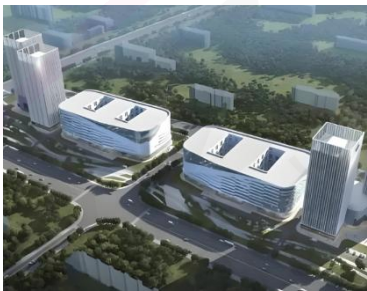
闽鲁智能港产业园幕墙工程, 济南, 山东 Minlu Intelligent Port Industrial Park, Curtain Wall Project, Jinan, Shandong
