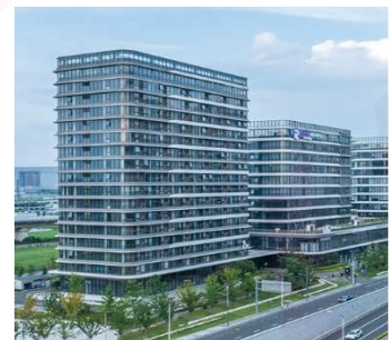
智高商务广场幕墙工程, 苏州, 江苏 Zhigao Business Plaza, Curtain Wall Project, Suzhou, Jiangsu
